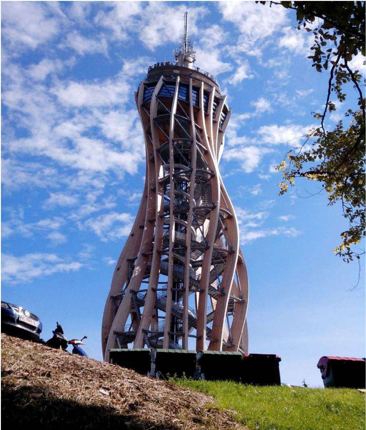
A 120 m high observation tower made entirely of wood
